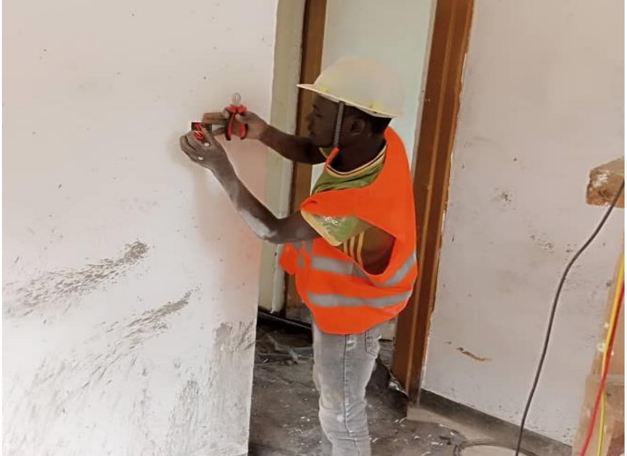
Figure 8 Young person doing wiring
